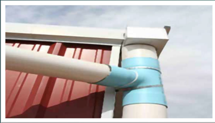
Rainfall is piped from the gutter
